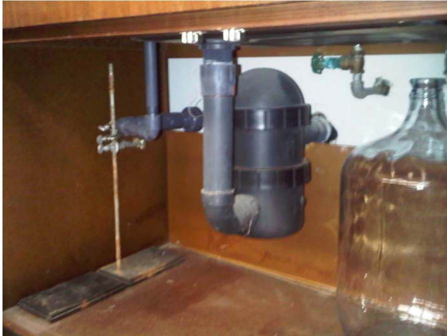
Sink trap with separator chamber. Remove piping to wall.
