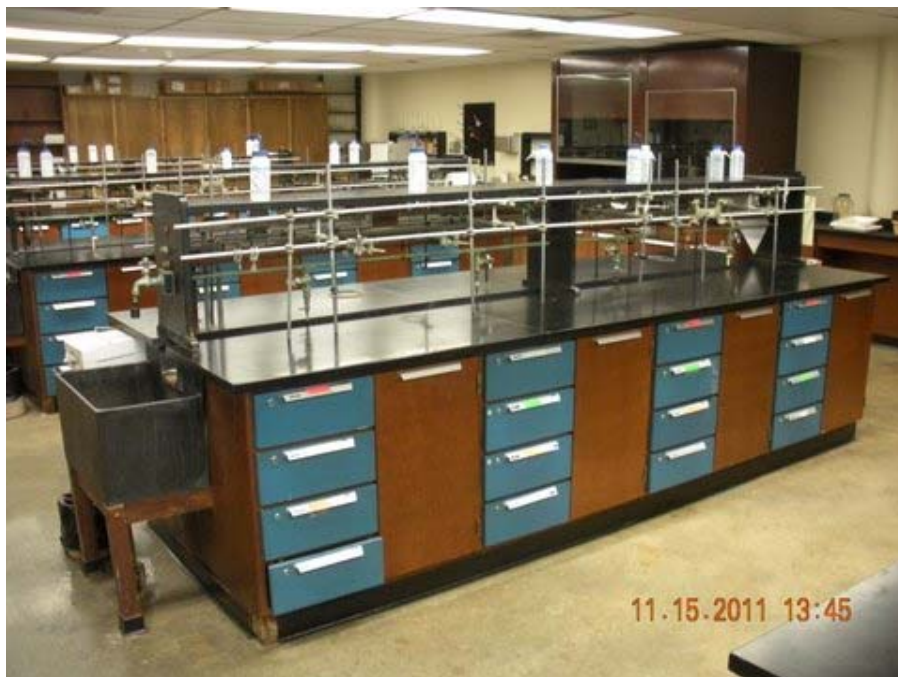
Lab benches with center trough, shelf, gas, water, electric and two sinks, Typical in chemistry labs
